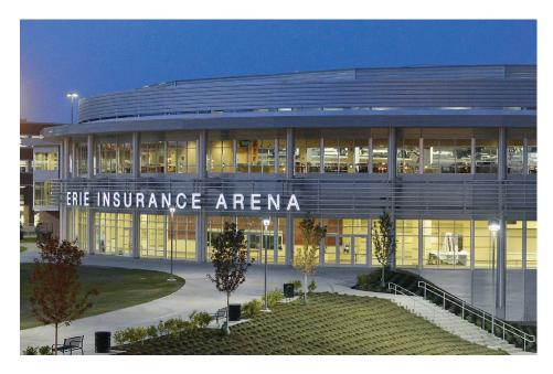
Renovations and improvements to Erie Insurance Arena included the addition of arena seating and significant enlargement of circulation areas, which increased the size of the arena from 152,000 square feet to a total area of 218,000 square feet, and boosted seating capacities to 6,500 for hockey, 6,750 for basketball and nearly 9,000 for concerts.
